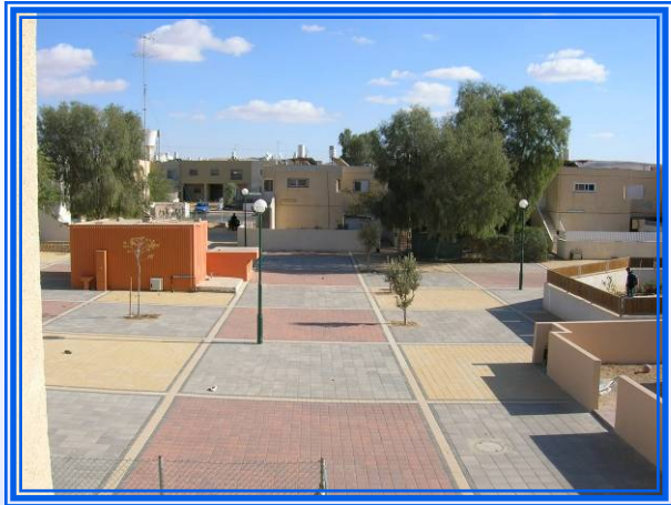
There are no streets in our neighborhood, only clusters of houses built around courtyards. Here's the view from our front door, looking down on the courtyard
